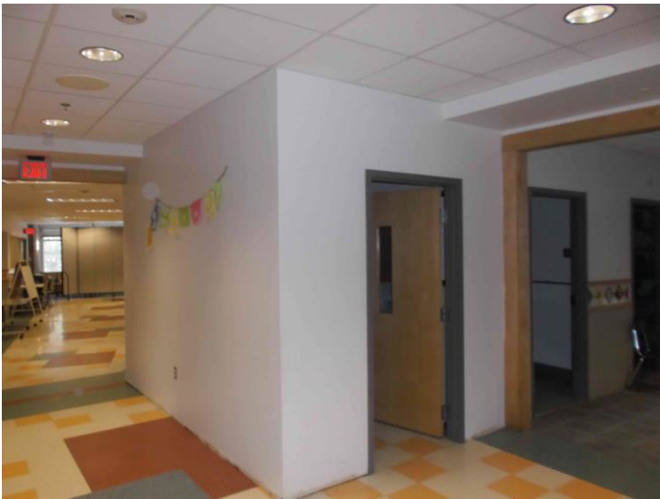
Additional offices and small meeting spaces have been created in hallways, and in part of the main office.
