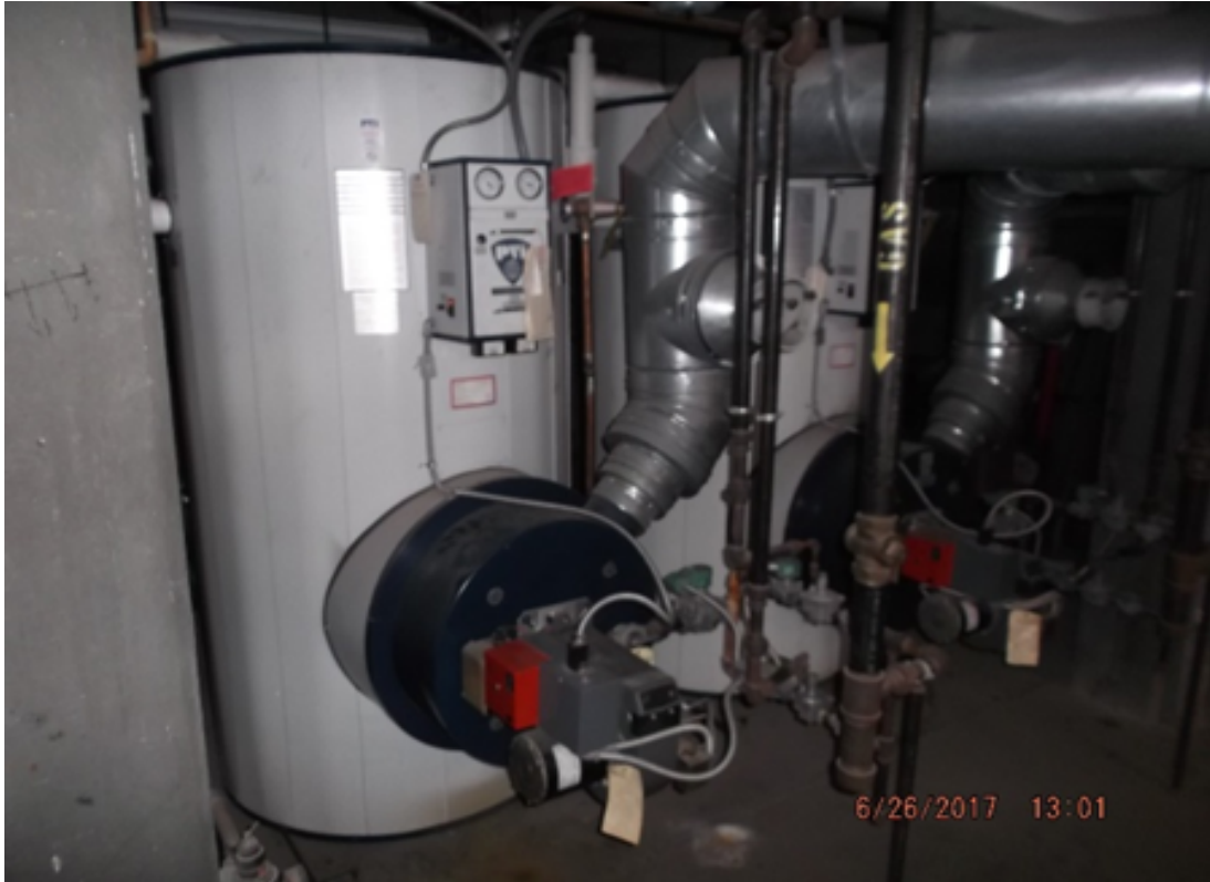
Old Gas-Fired Hot Water Heater (above) replaced with Electric Hot Water Heaters (below)
