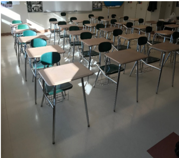
Old 12"x12" VCT (vinyl composite titles) replaced with low maintenance and more durable VQT (vinyl quartz tiles) at John Glenn Middle School.
