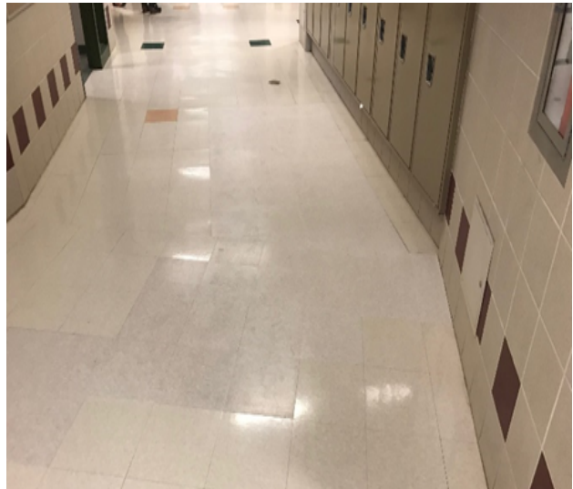
Old 12"x12" VCT (vinyl composite titles) replaced with low maintenance and more durable VQT (vinyl quartz tiles) at John Glenn Middle School.
