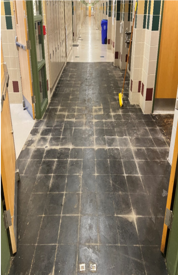
Old 12"x12" VCT (vinyl composite titles) replaced with low maintenance and more durable VQT (vinyl quartz tiles) at John Glenn Middle School.
