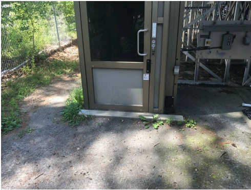
Figure 10 – Granite curb at HC Lift
