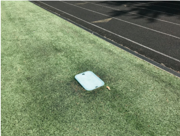
Photo 13 - Turf Field - Irrigation Handhole
