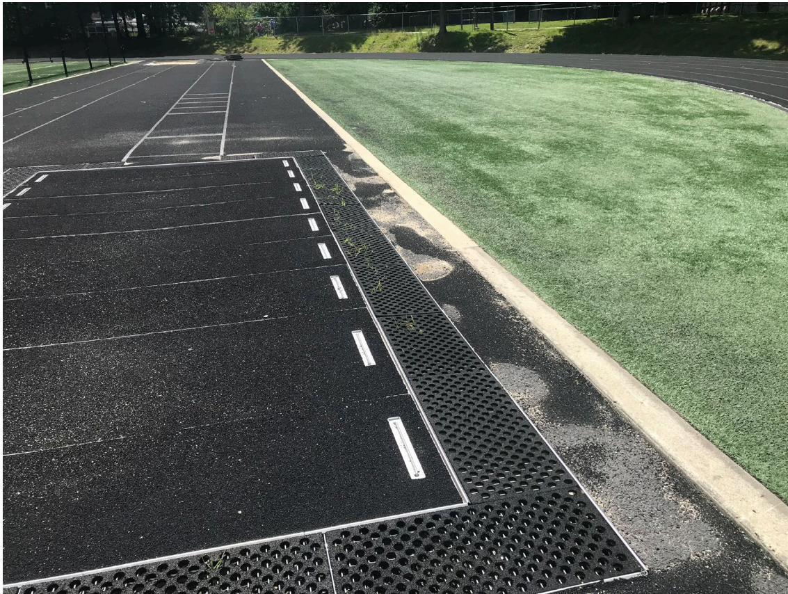
Figure 4 – West ‘D’ Area – Asphalt Settlement
