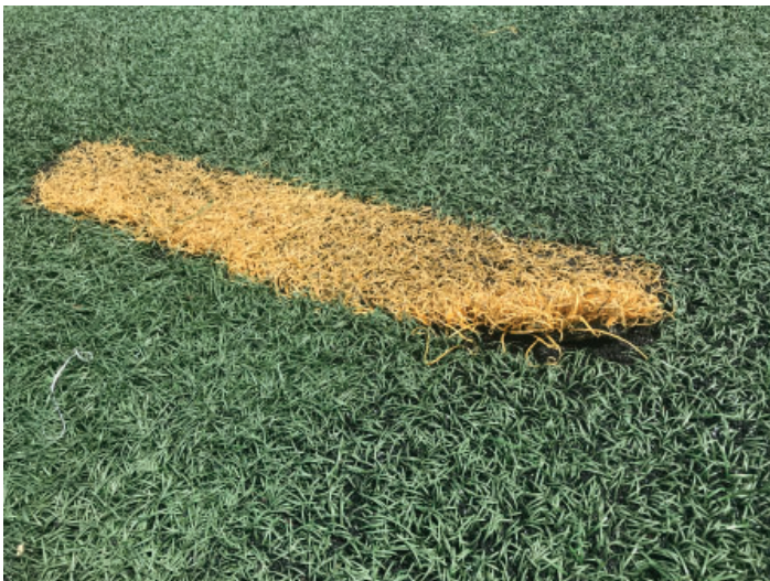
Photo 17 -Turf Field - Loose Seam
