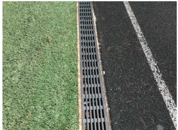
Photo 18 - ACO Trench Drain - Full of Debris
