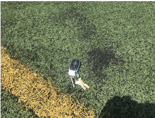
Figure 8(a) – Fiber wear & exposed infill
