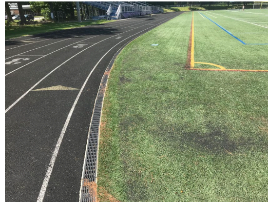
Figure 8(b) – Fiber wear & exposed infill
