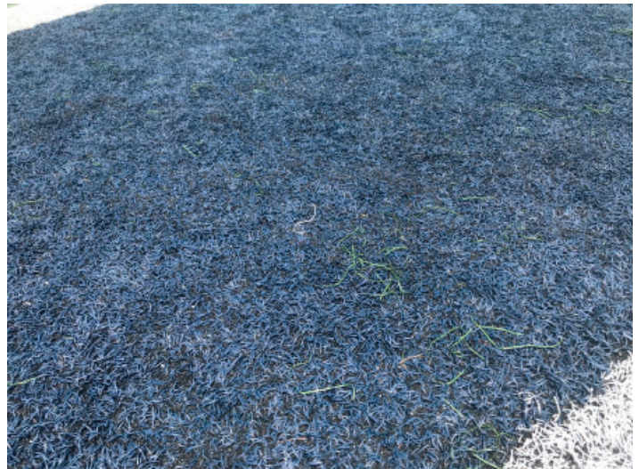
Photo 16 - Turf Field - Loose Fiber
