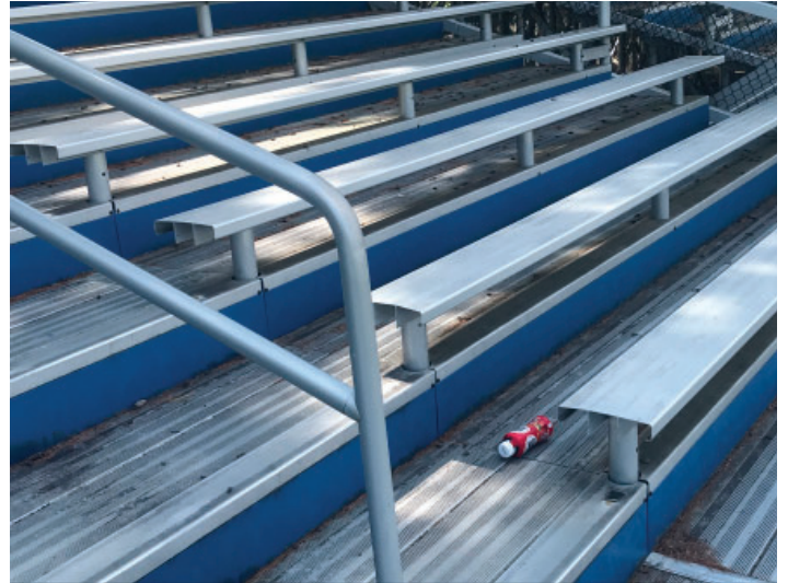
Photo 26 - Existing Home Bleacher - Missing End Caps
